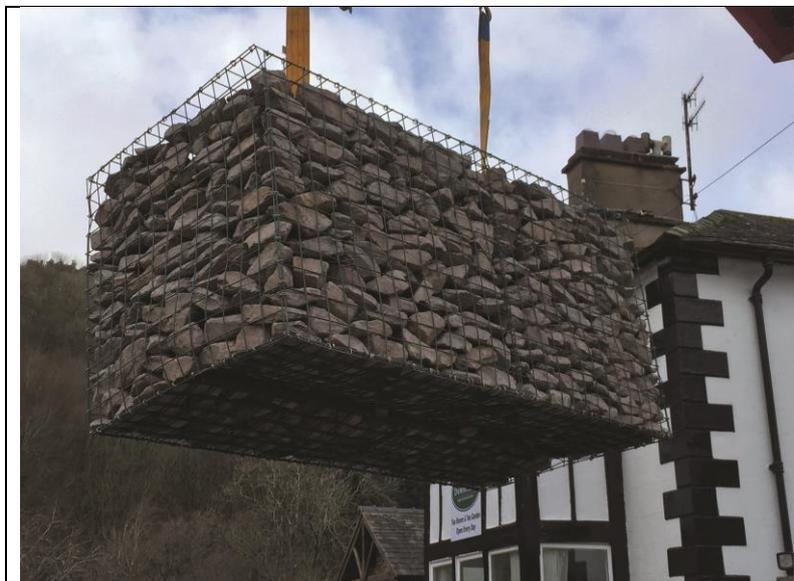
11.11 Purpose-made lifting frames and slings must be used for lifting filled units which weigh up to 1.8 tonnes per cubic metre (see Figures 10 and 11).
