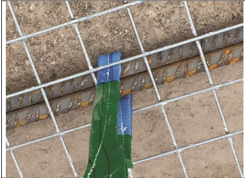
*Figure 11 Gabion filled and braced as normal, with lifting strop/chain vertical*
