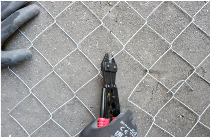
**METHOD A - Step 2:** Grab a mini bolt cutter and cut the marked strand from bottom to top.
