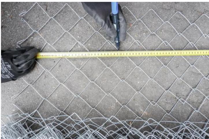
**METHOD B - Step 1:** To make sure you follow the same strand when unhooking the ends, mark along the length of the strand where you'd like your first section to end.
