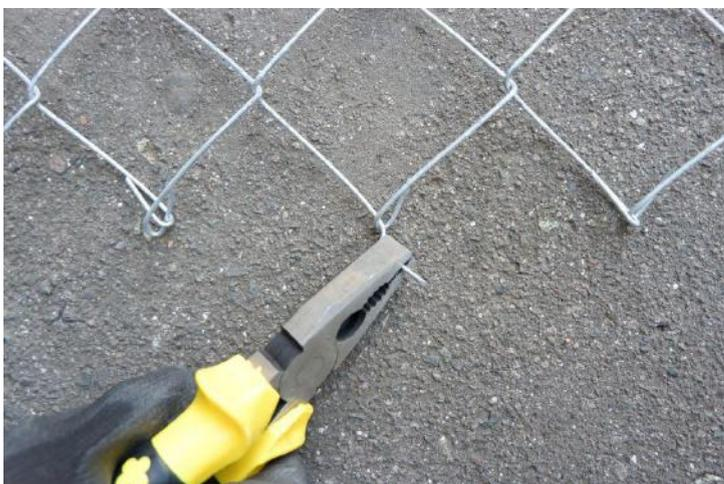
**METHOD B - Step 2:** Use a plier to unhook the top and bottom ends of the strand you just marked.
