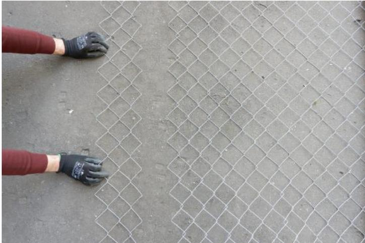
**METHOD A - Step 4:** After you're done removing the offcuts, pull the separated section away from the rest of the roll.
