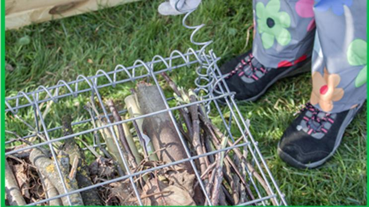
Close the lid, ensuring it sits comfortably on the fillings without any gaps. Secure the top around the edges with the helicals, using the same technique as before.
