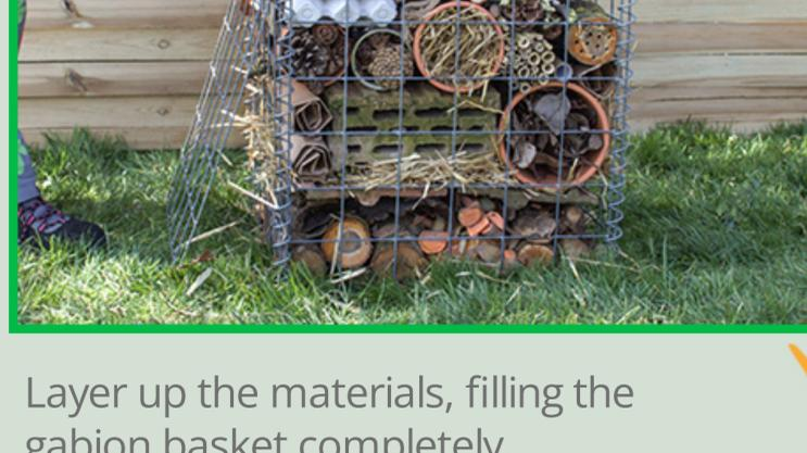
Layer up the materials, filling the gabion basket completely.
