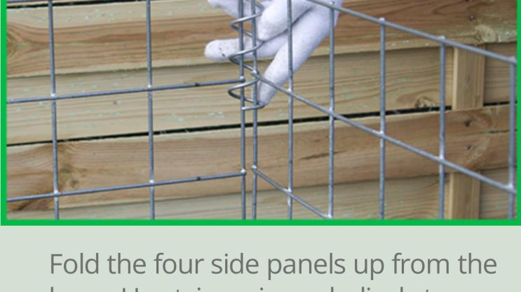
Fold the four side panels up from the base. Use tying wire or helicals to attach the corners. If these aren't available, cable ties or rope can serve the same purpose. Twist the helicals into place, ensuring they secure the corners of both panels.
