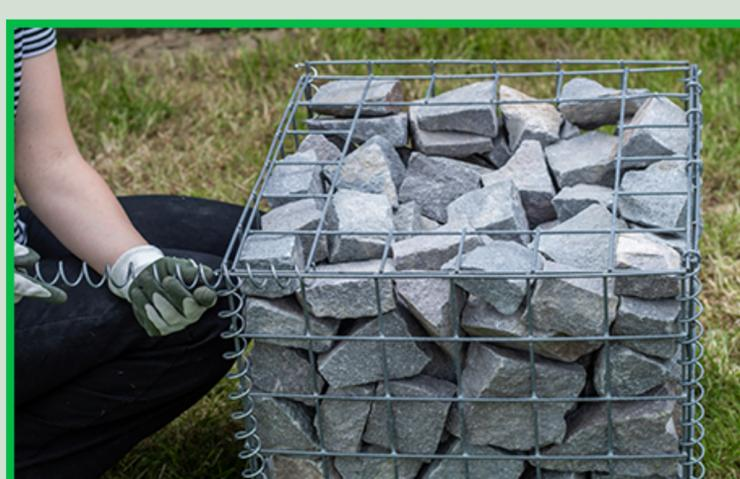
Use the helicals to secure the top around the edges, ensuring a snug fit and that all rocks remain in place.
