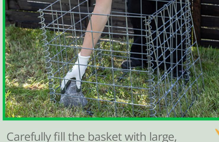
Carefully fill the basket with large, durable, non-degradable rocks that are larger than the mesh aperture.
