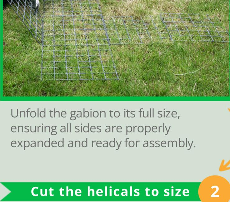
Unfold the gabion to its full size, ensuring all sides are properly expanded and ready for assembly.
