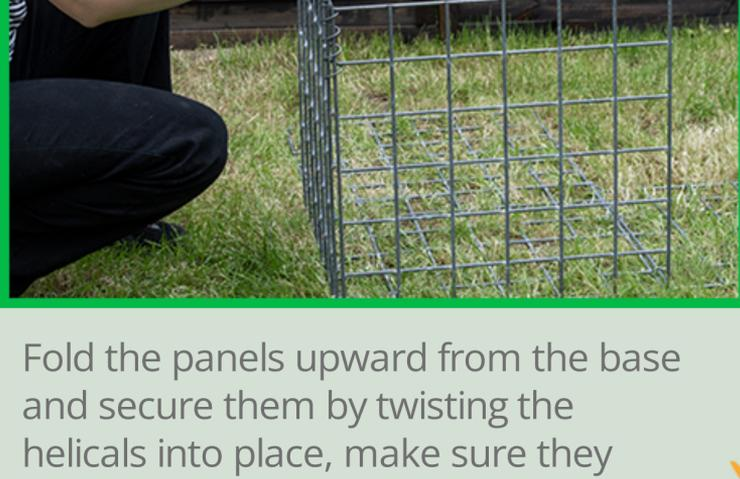
Fold the panels upward from the base and secure them by twisting the helicals into place, make sure they encompass the corners of both panels. Repeat this process for all panels while leaving the lid open.
