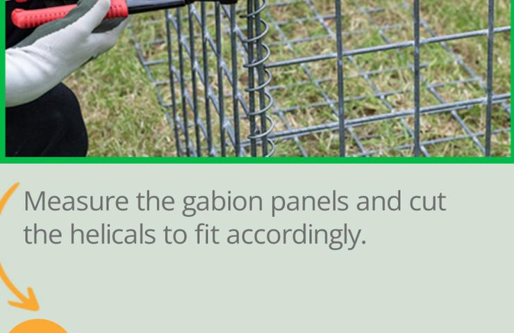
Measure the gabion panels and cut the helicals to fit accordingly.
