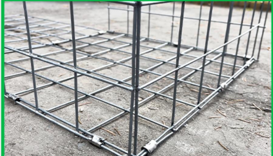
Inspect the gabion for remaining bends or irregularities, ensuring the wire is intact.
