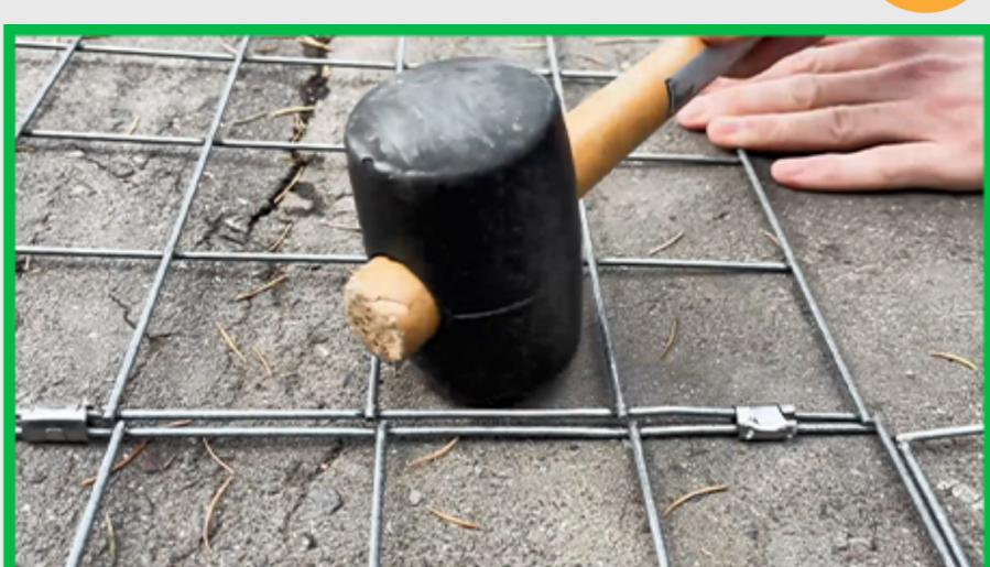
Continue this process on each side of the gabion, gently knocking it back into shape wherever it is bent.
