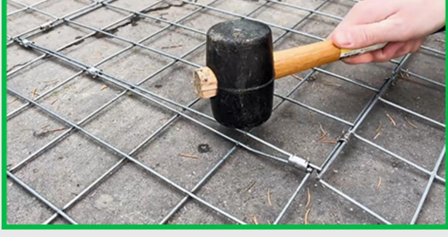
Place the gabion on a solid surface and carefully tap it back into shape using a rubber hammer.
