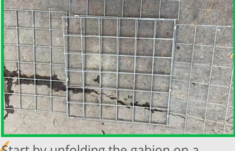
Start by unfolding the gabion on a stable, solid surface to ensure proper support while working.
