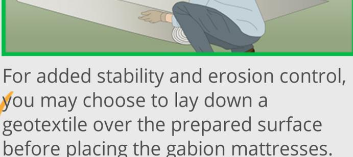
For added stability and erosion control, you may choose to lay down a geotextile over the prepared surface before placing the gabion mattresses.
