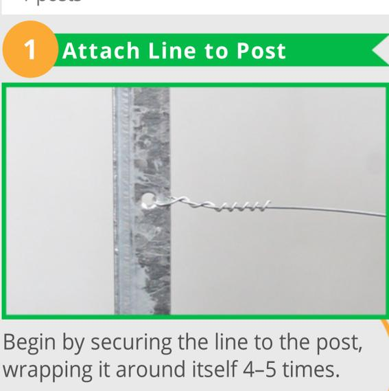
Attach the line to the post by placing it in the hole, then wrap it around itself 4-5 times to maintain the tightness.
