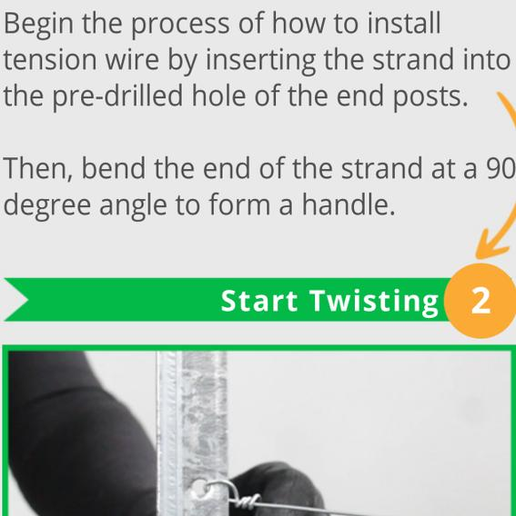
Begin the process of how to install tension wire by inserting the strand into the pre-drilled hole of the end posts.
