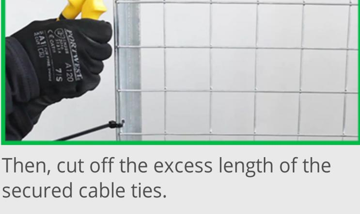
Then, cut off the excess length of the secured cable ties.
